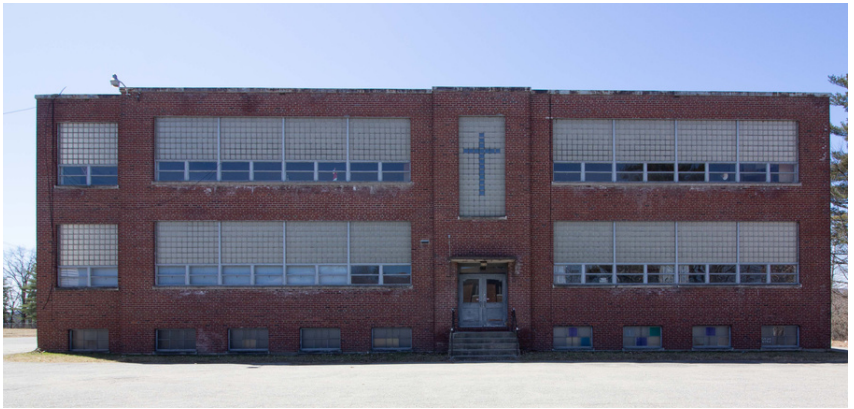
A vacant Sacred Heart School building in 2023
